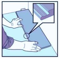
Be sure to install the first row of boards with the tongue side facing the wall. See diagram on left.
